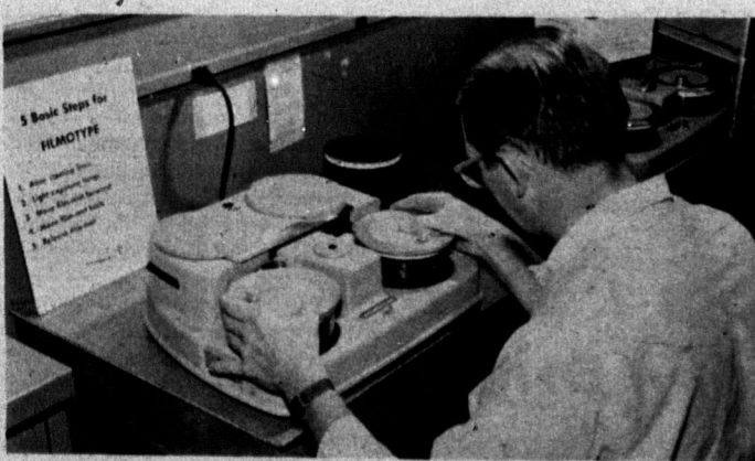
Fotosetter , one of several phototypesetting machines, externally resembles its hot metal counterpart, the Intertype slug-casting machine. But in place of the traditional metal pot, a camera is used. The operator has a choice of eight type sizes from a single photographic matrix. Lines of type are produced on sensitized paper or film instead of metal. ITU Training Center Instructor Alex Coleman, seated, explains it all to ANG President Arthur Rosnstock, left, Executive Vice President William J. Farson, center, and Director of Research and Information Ellis T. Baker.
