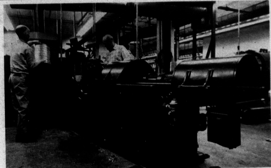
Expediter: Latest installation at the nearly-completed plant of The Portland Reporter is this factory-rebuilt semi-automatic plate caster. It enabled the staff, union members on strike
