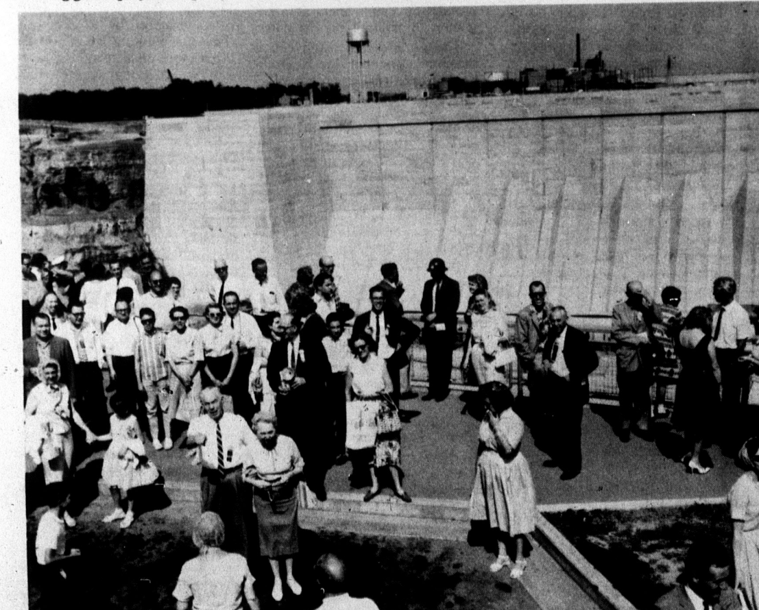
MASSIVE FACING of the Robert Moses Niagara Power Plant, housing thirteen 24-foot penstocks leading to turbine generators, is seen from the Canadian side of the lower gorge, where the Sir Adam Beck generating plant shares the river's power potential with the United States.
