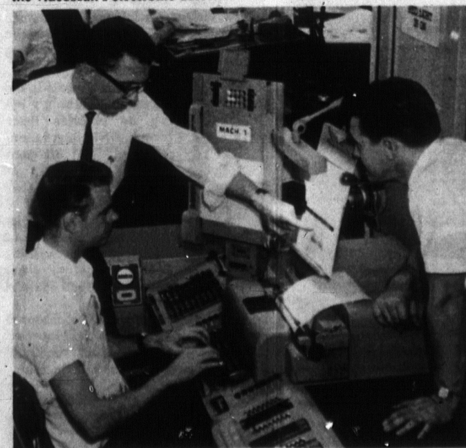
VERSATILE PERFORMER: An operator punches the keyboard of one of the Chicago Sun-Times and Daily News' four new electric photocomposition machines, which set and make up ads. A management spokesman says they can be adapted to editorial uses in the future, as well.
