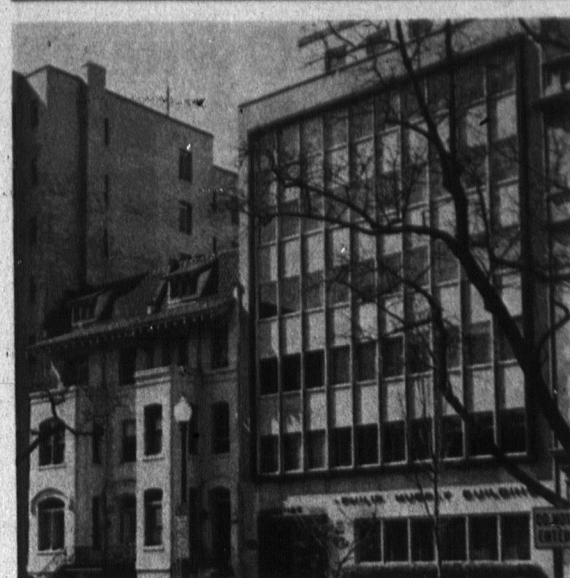
EXPANSION: The IUE's Philip Murray Building, in which ANG headquarters occupies a floor, is being doubled in size. The structure at left, above, has been torn down to clear space for erection of the addition. At right, how the Washington building will look when construction is completed late next year.
