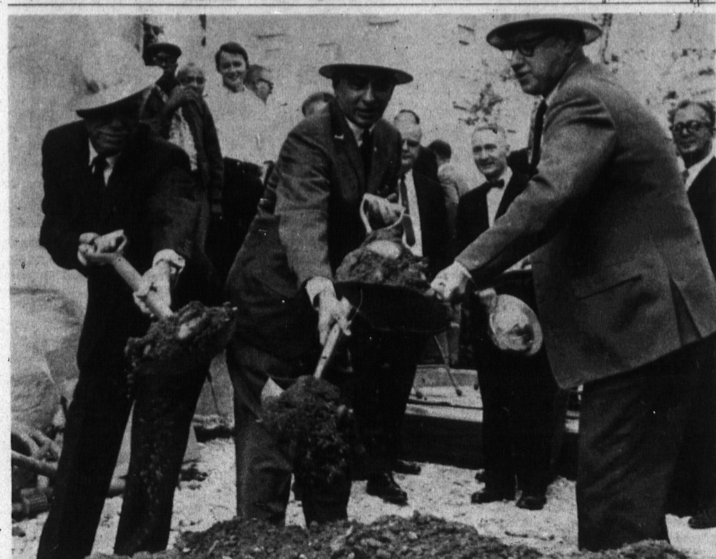
BREAKING NEW GROUND: ANG Executive Vice President William J. Farson, left, joins IUE President James B. Carey, center, and Victor Reuther, administrative assistant to UAW President Walter P. Reuther, in turning the first shovelful of earth for a $1.5 million addition to the IUE's Philip Murray Building in Washington, where ANG international headquarters are located. It will double the building's size when completed late next year.
