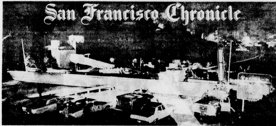
Early yesterday a dump truck full of dirt knocked down a pedestrian overpass on the James Lick freeway at 18th street. The dump section of the truck, behind the fallen overpass at the left, shot into the air, hit the walkway and brought the whole thing tumbling down. The truck tractor stopped 100 feet ahead. Another picture and story on Page 9.
