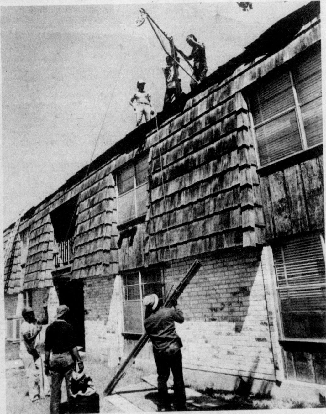
REPAIRS PROCEED AT SAN ANTONIO GUILD PARK APARTMENTS Workers prepare to hoist a gravel guard to a roof.
