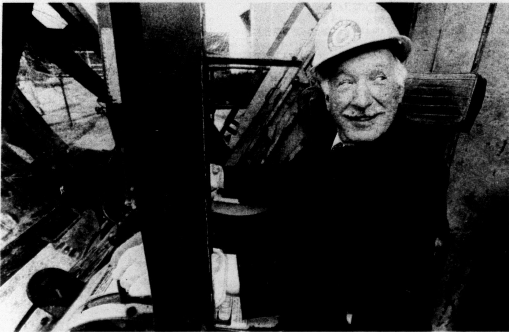
JOSEPH E. COLE DIRECTS WRECKING BALL INTO OLD CLEVELAND PRESS BUILDING Cleveland industrialist cleared site late in 1983 for new office complex.
