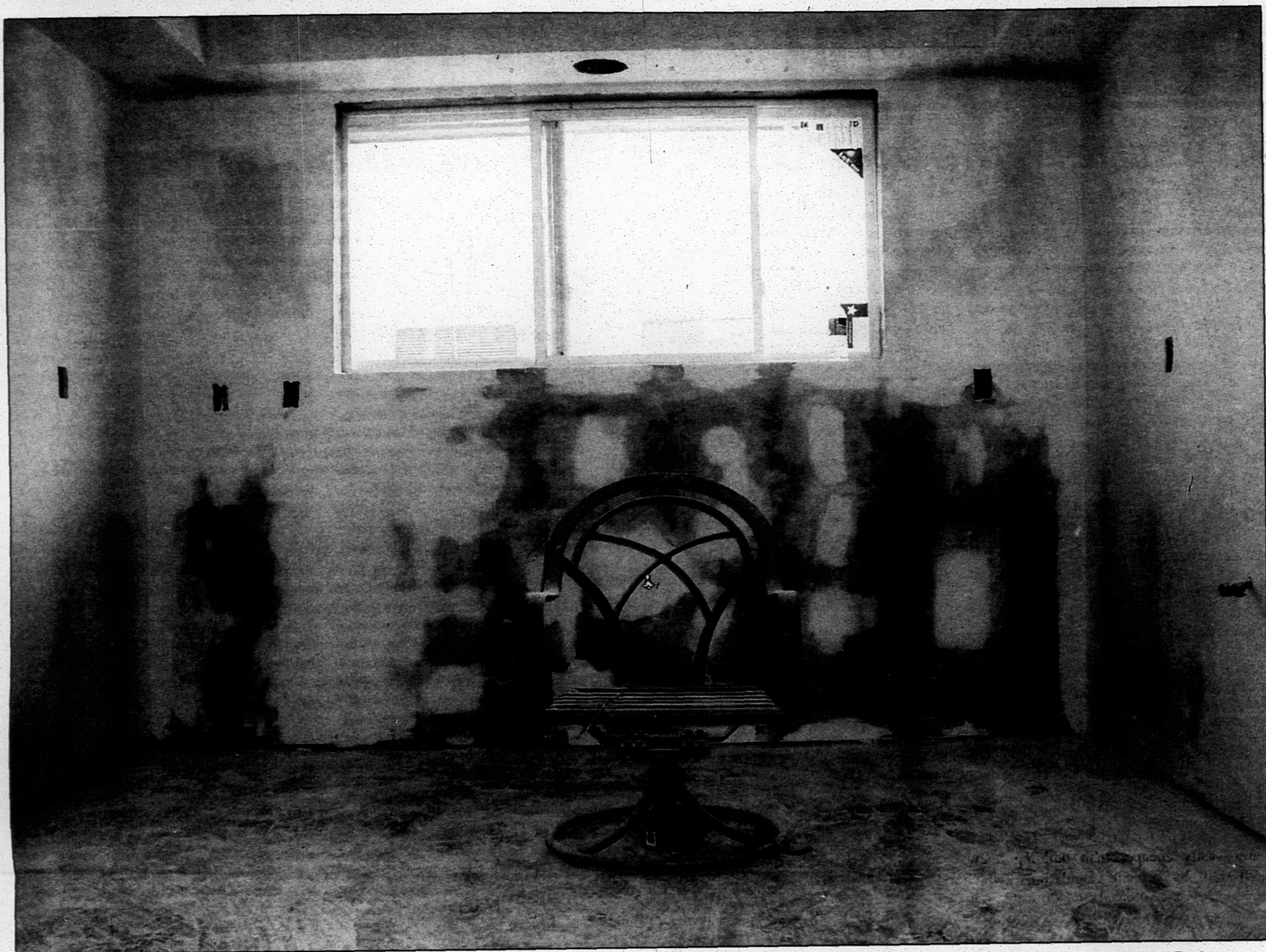
A steel-framed chair, the only piece of furniture Sidney and Joe Navis were able to rescue, sits in a room of their house as it's being repaired by the St. Bernard Project.
